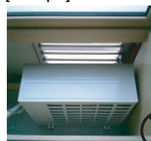
<Without air guide> Safety device activation
